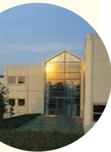
Fire risks have been minimised in the projecting and layout of buildings.
